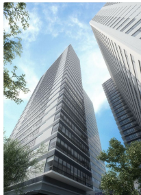
Vista inferior del edificio Lower view of the building
