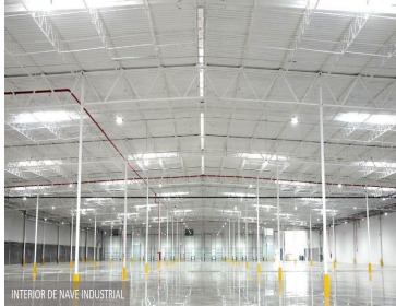
INTERIOR DE NAVE INDUSTRIAL
